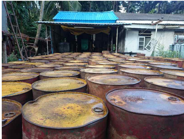
Figure 5 Drums full of diesel stacked up at a diesel generator at Havelock Island, India [6]
